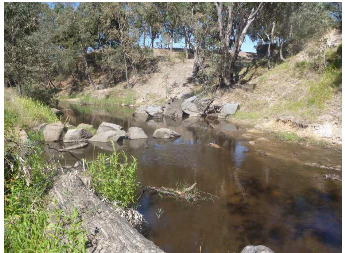
Past reinstated structures in Seven Creeks downstream of Galls Gap Road
