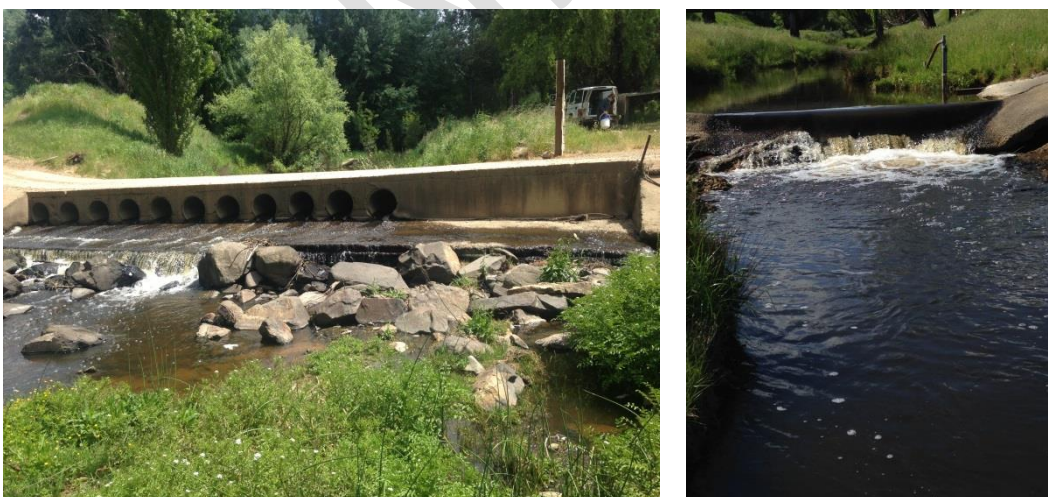
Figure 3. Barriers to fish passage hinder habitat connectivity and restrict fish access to refuge areas. a) Brankeet Creek at Mitchells Road, b) Brankeet Creek at gauging station downstream Lonergans Road.
