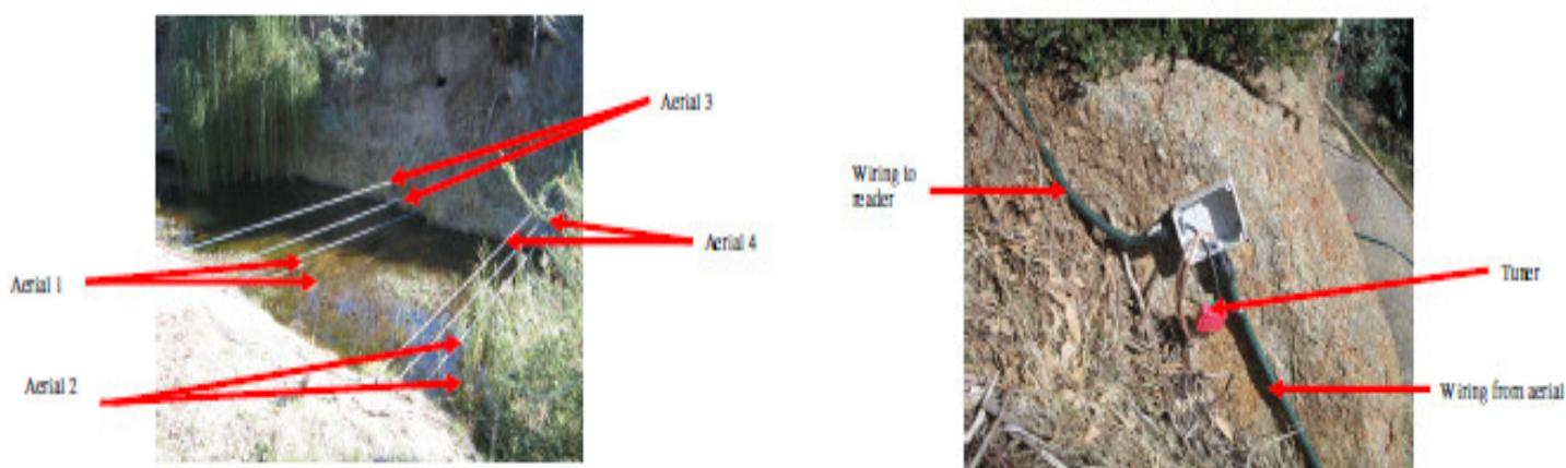
Figure 2 PIT tag wiring and aerials present 1km upstream of Galls Gap Road Bridge.
