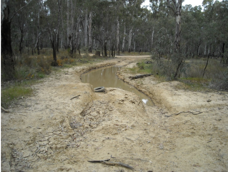
Figure 18 Vehicle access in wet conditions has led to the development of ruts in riparian reserves. Tracks with poor drainage and clay bases appear to be more susceptible
