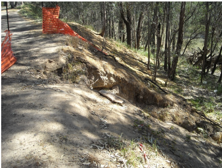
Figure 17 A small section of piping erosion observed adjacent to Aquamoves on the right bank of the Goulburn River
