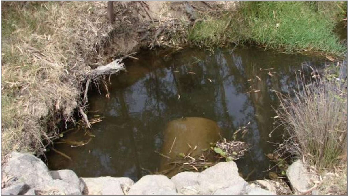
Figure 1. Pipe culvert beneath the main Tahbilk road crossing.
