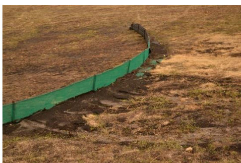
Figure 3: An effective silt fence after recent rains in the fire affected area
