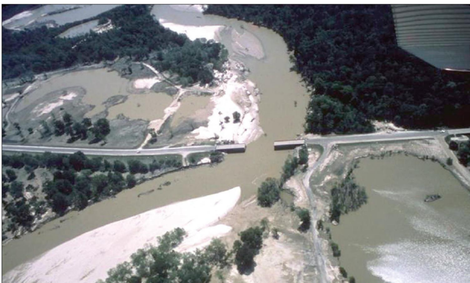
Figure 2.3 : Looking downstream to the bridge failure at State Highway 10 near Arcola along the Tangipahoa River in Louisiana, USA. Mossa and Marks (2011) attribute this bridge failure to mining related degradation.
