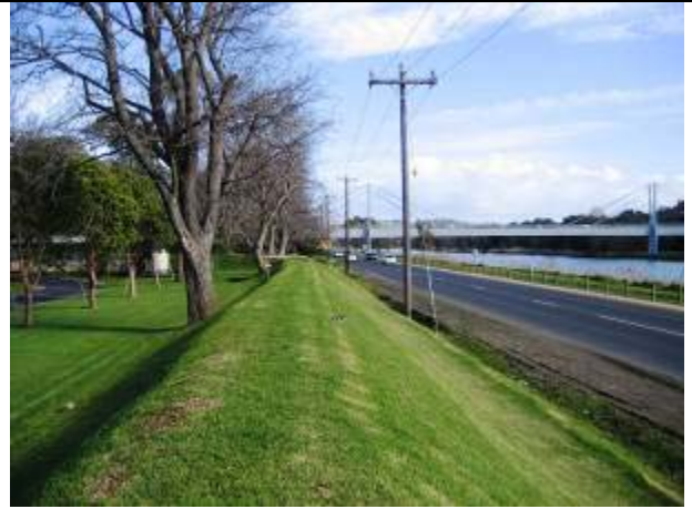
b. Levee around caravan park (Corangamite CMA)
