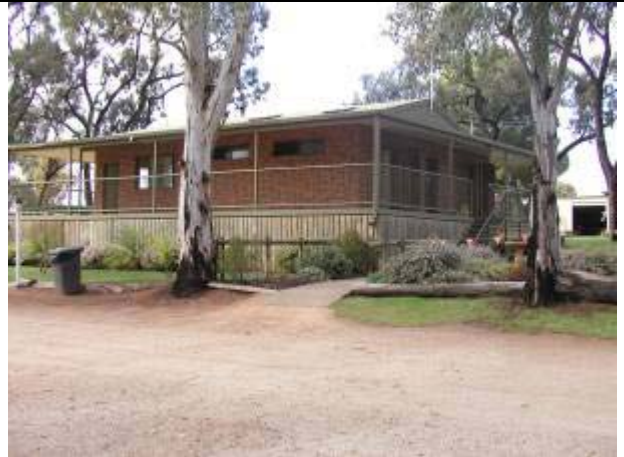
h. Raised amenities block, above 1956 flood level (Mallee CMA)
