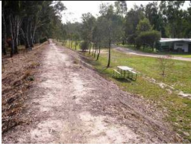
a. Levee around caravan park (Goulburn Broken CMA)
