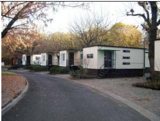
e. Raised cabins, to 1993 flood level (North East CMA)
