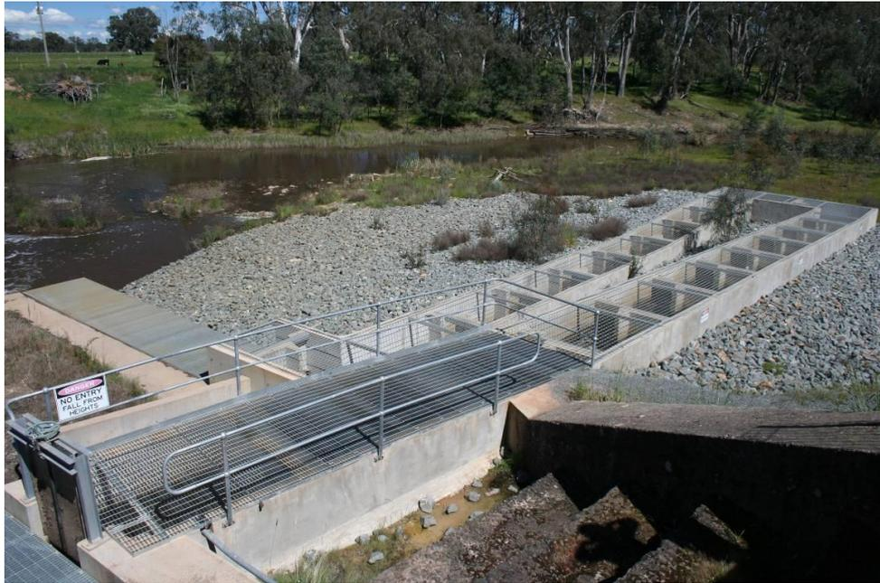
**Figure 2.** Vertical slot fishway on Casey's Weir. Photo: Rick Stoffels.
