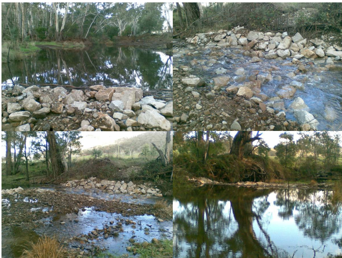
Slide 4. Construction of rock-bar at McCauleys Crossing.
