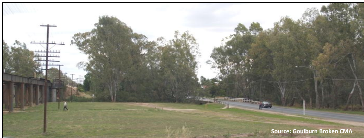
Photo 5: Stock Bridge (Ackerly Avenue) across the Broken River floodplain. Railway viaduct shown in the left
