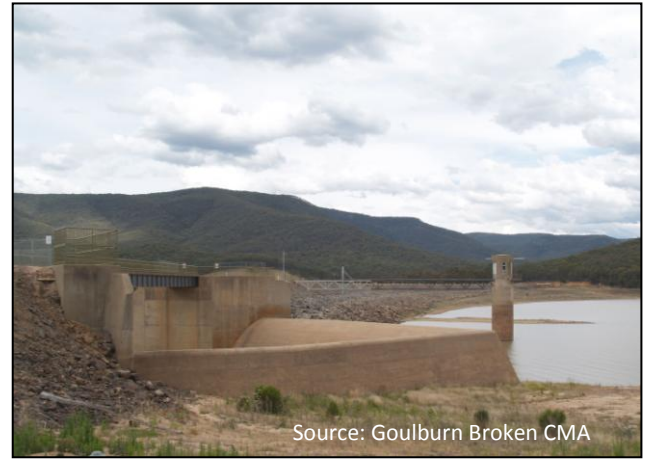
Photo 1B: Nillahcootie dam wall showing spillway
