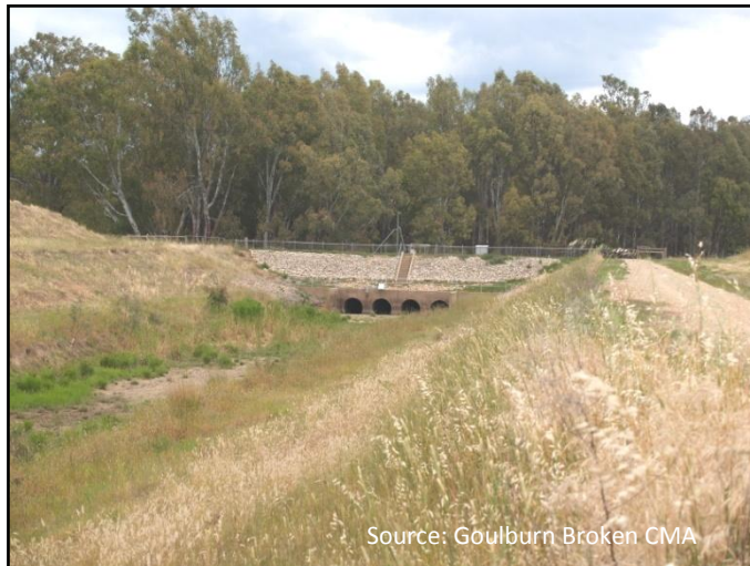
Photo 3: Mokoan inlet (diversion) channel from Broken River
