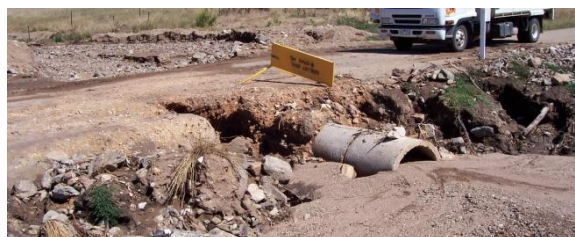
Above: A flash flooding event which eroded the road surface (source NECMA)
