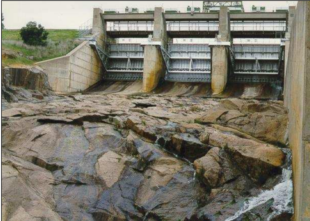
■ Figure 19 Cairn Curran Reservoir Spillway Gates
