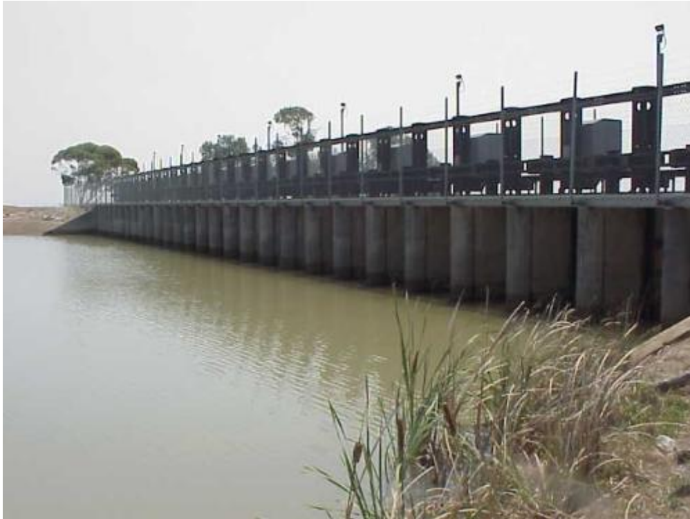
■ Figure 25 Loddon Weir – Looking at upstream side of structure
