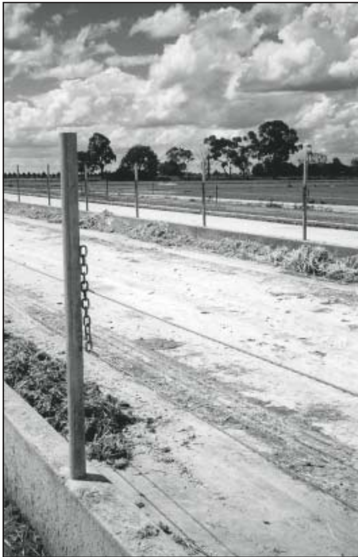
Figure 17: Concrete feedpad showing feed bay with cable and chain restraints.
