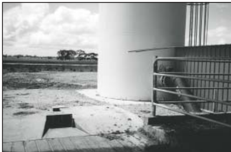
Figure 23: Flood washing tank and outlet.
