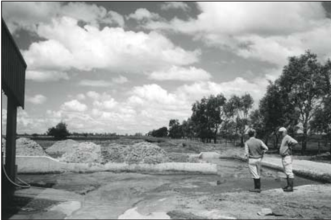
Figure 25: The solids trap at the end of the feedpad collects the sand and any remaining solids are removed in the long thin settling pond (in background) prior to effluent entering an effluent pond.
