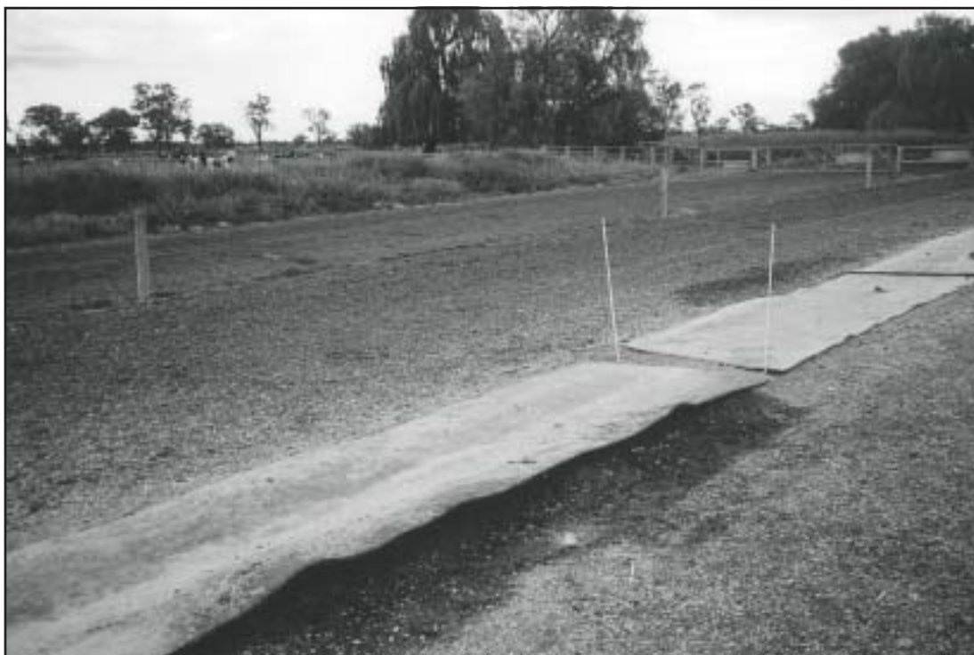
Figure 11: Conveyor belt lifting and pad surface breaking down - this is periodically patched up with additional rock.
