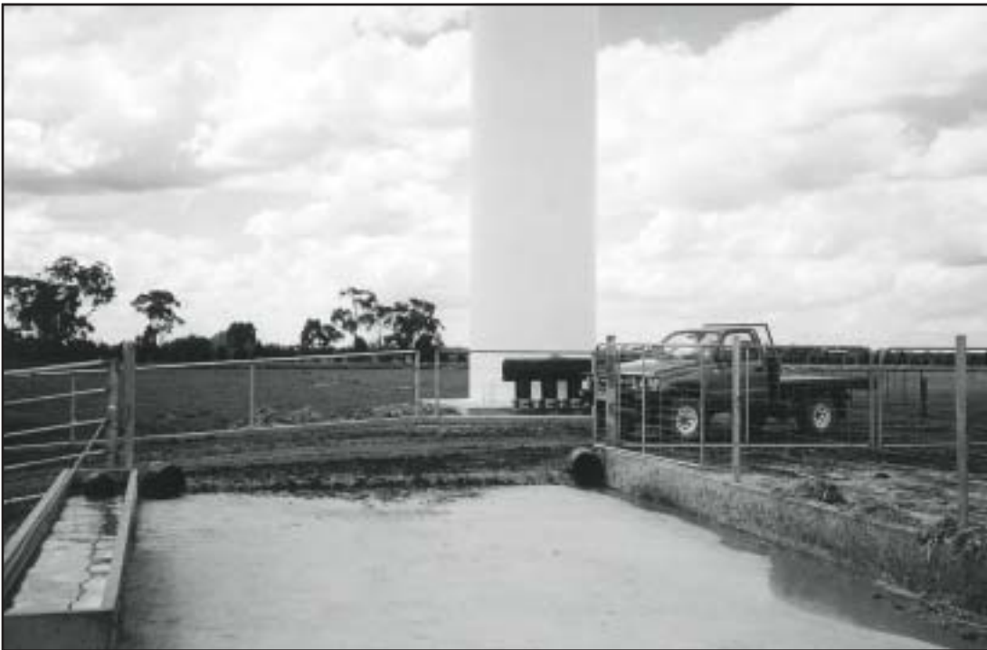
Figure 18: Drinking water trough, flood wash outlets and flood washing system tank at top of pad.
