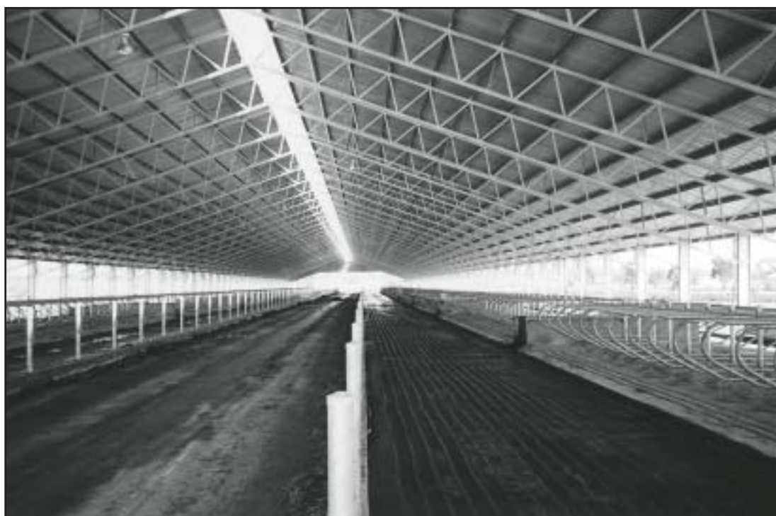
Figure 21: View from the bottom of the free stall barn. Feed bay on left, cow alley and cow stalls on right.
