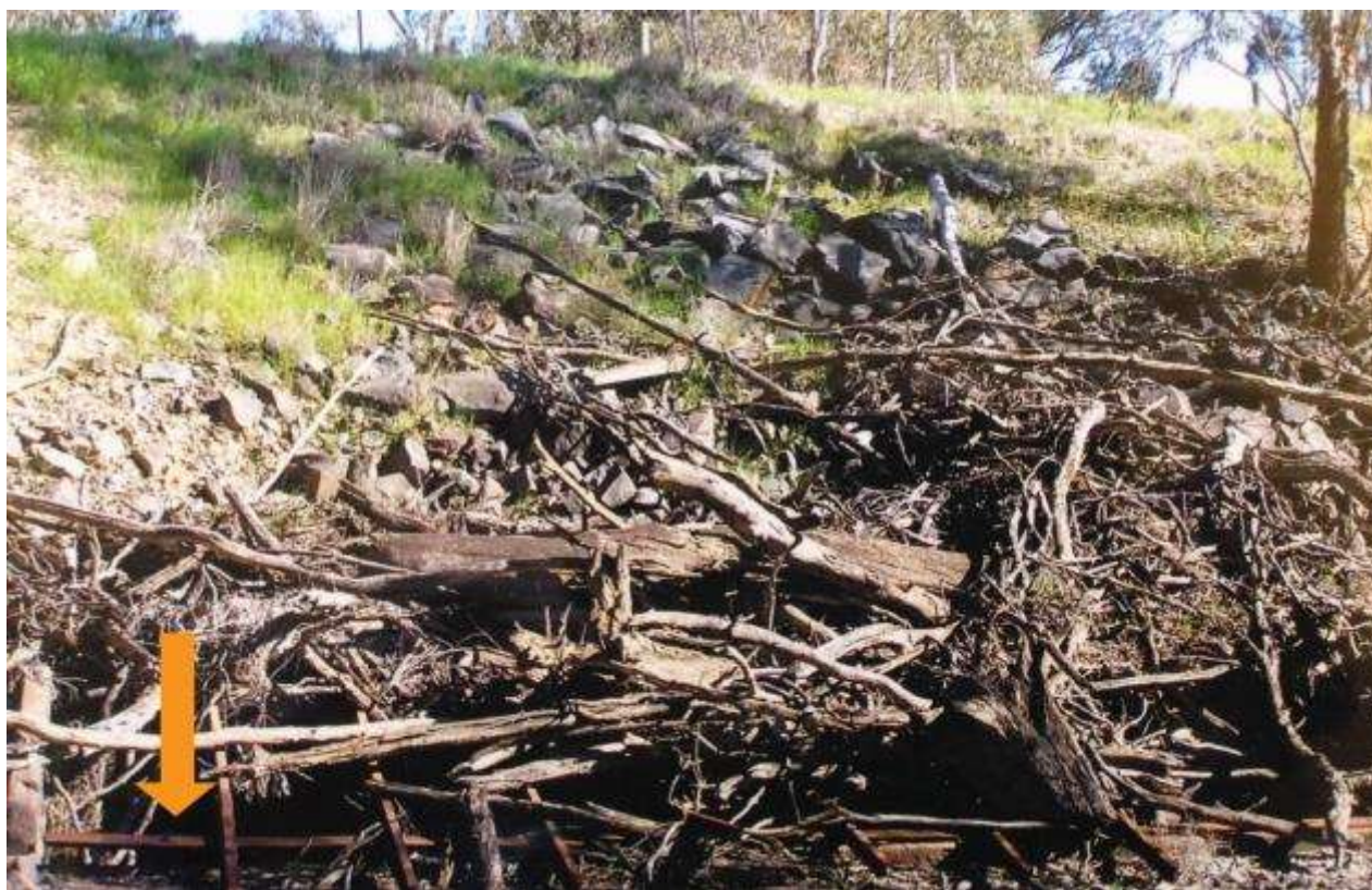
Hancocks pipes through the levee bank, almost completely clogged with debris (the arrow indicates the position of the pipe). Photo: Morris Brown
