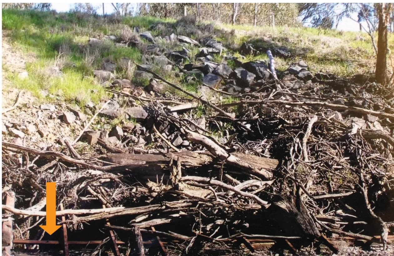
Hancock pipes through the levee bank, almost completely clogged with debris (the arrow indicates the position of the pipe). Photo: Morris Brown
