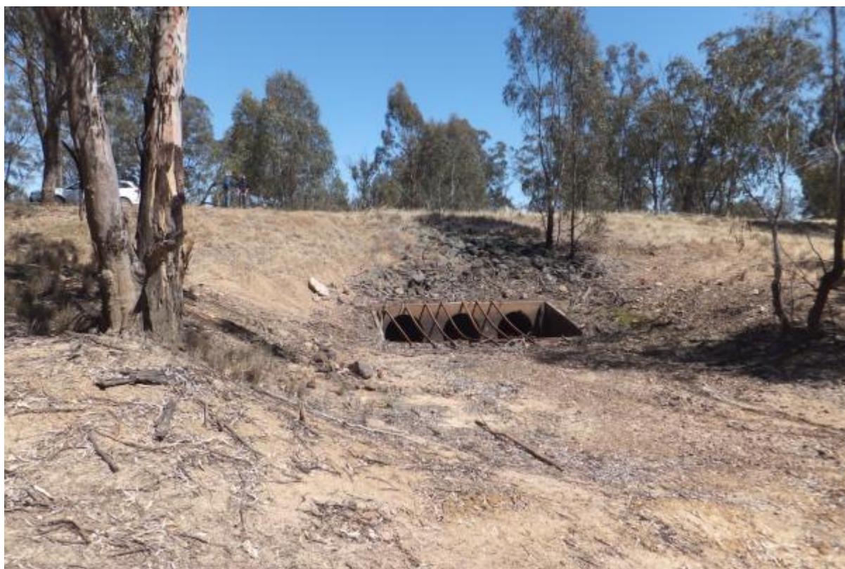
Hancocks pipes through the levee bank after debris has been removed. Photo: Geoff Earl, GB CMA
