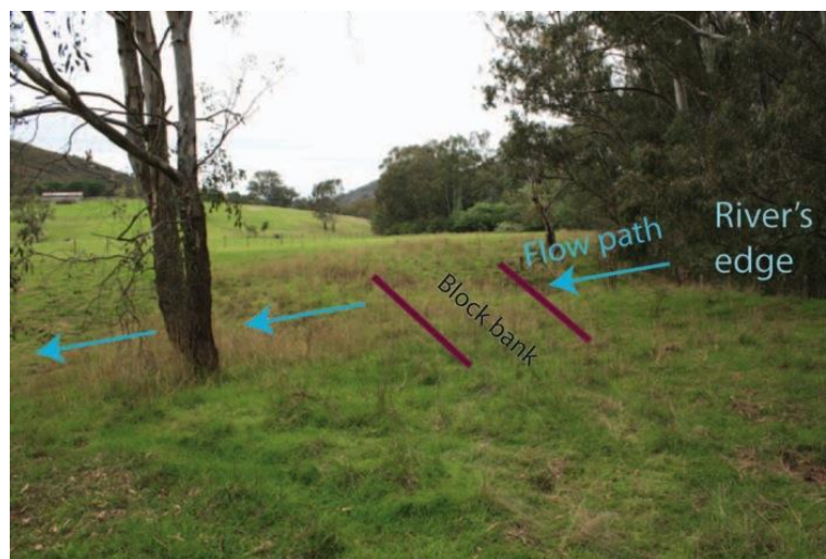
Figure 14: Block bank reducing inflows to a flood runner immediately upstream of Horseshoe Lagoon (Reach 2). (Photo: Geoff Vietz).
