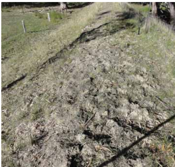
Erosion : rilling (below)
