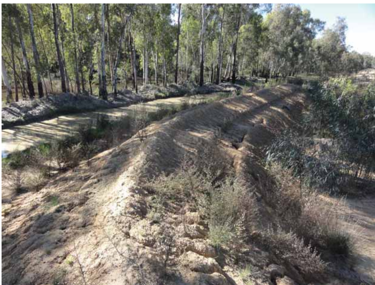
Erosion : rilling (below)
