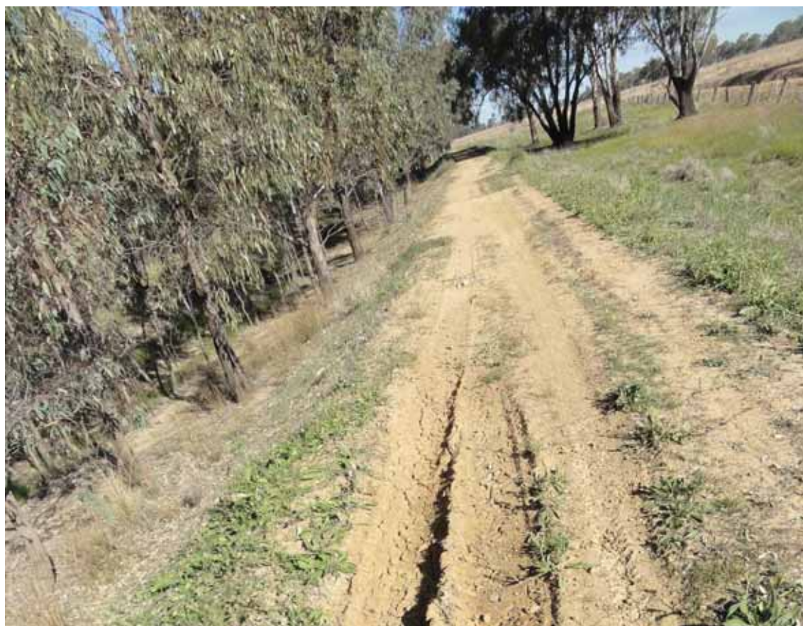
Hole : sink hole (above); Hole : wheel ruts (below)
