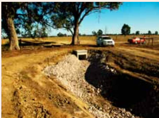
The boring under trees policy was implemented for the first time during construction of the Muckatah 4P community surface water management system. Photo: John Bourchier, DPI
