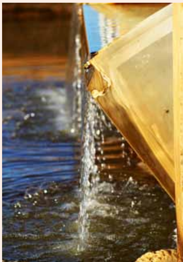
Water over a flume gate regulator. Photos: Chelsea Nicholson, DPI
