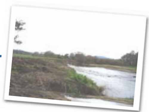
Willows cleared in preparation for native revegetation
