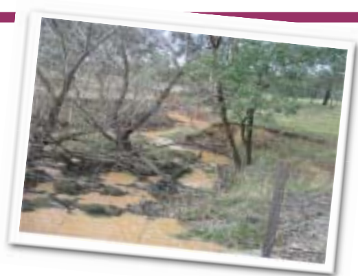
Silt delivered from an eroded tributary.
