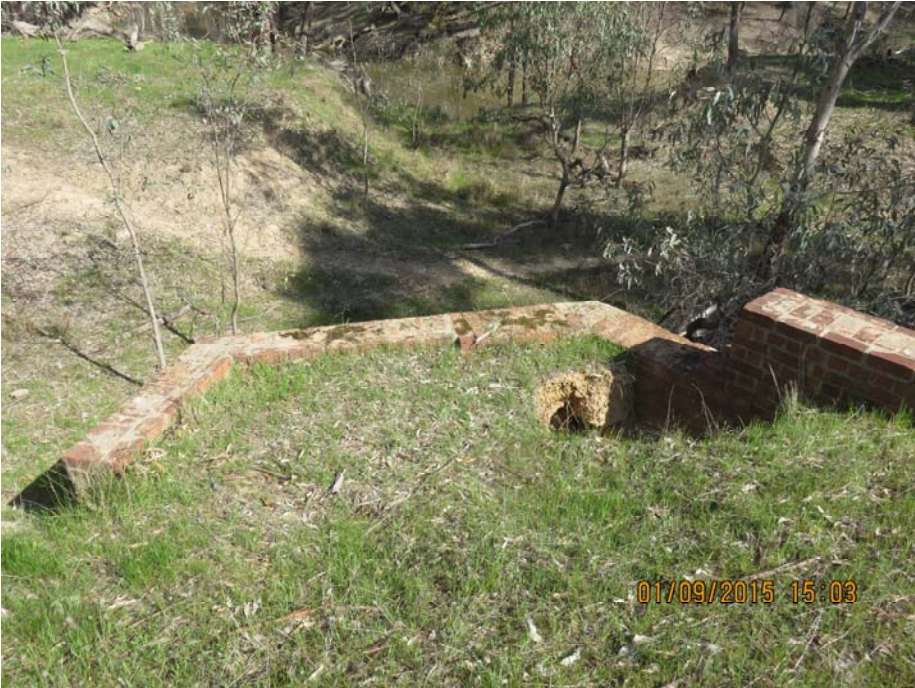
PHOTOGRAPH No.30. Subsidence behind wall above missing shelf.
