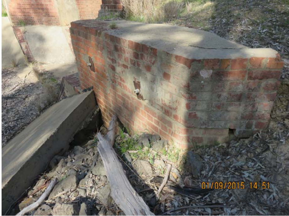
PHOTOGRAPH No.4. Note back of wall has been backfilled with mass concrete.
