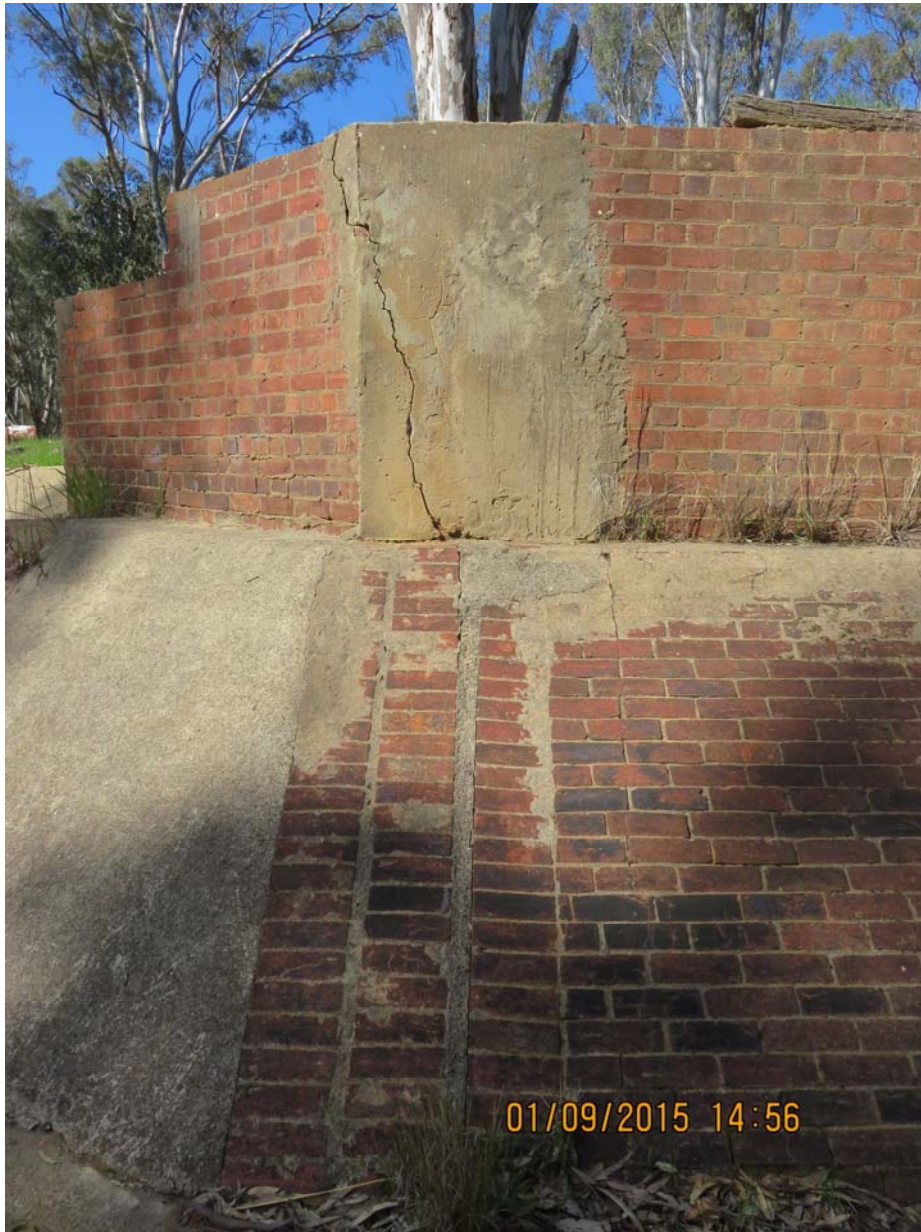
PHOTOGRAPH No.29. Vertical crack.
