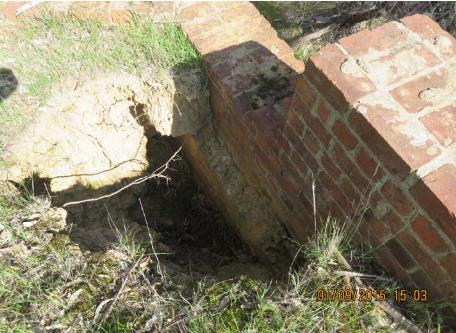
PHOTOGRAPH No.31. Subsidence is more than 1.2m deep.
