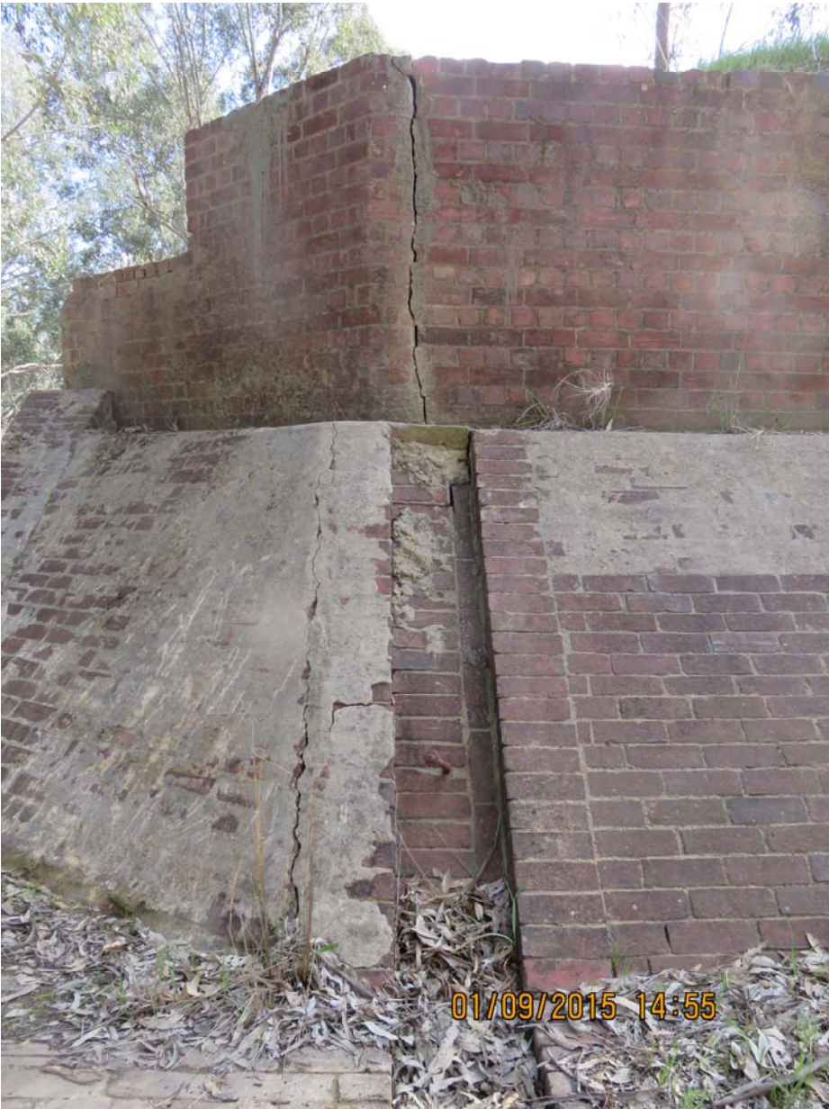
PHOTOGRAPH No.46. Note vertical crack in west abutment on upstream side.
