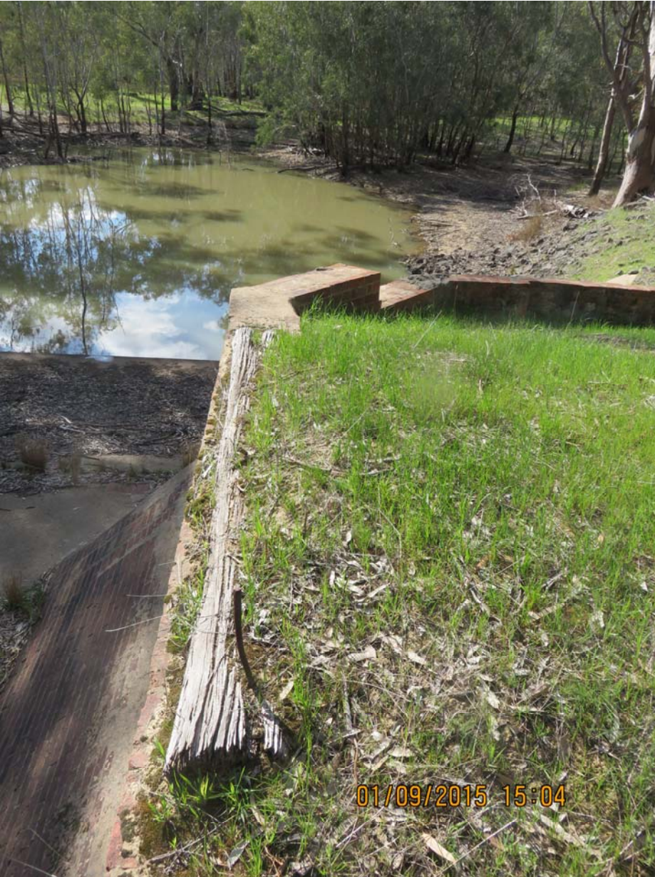
PHOTOGRAPH No.32. Note remnants of timber bridge deck.
