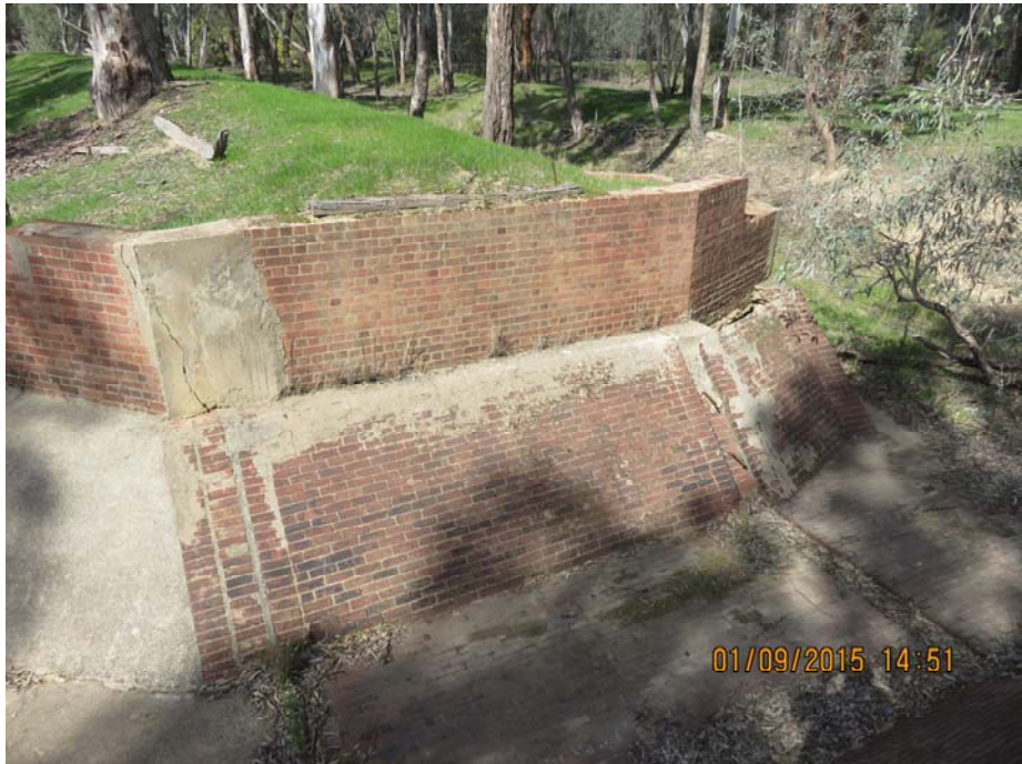
PHOTOGRAPH No.28. Note vertical crack on downstream side.
