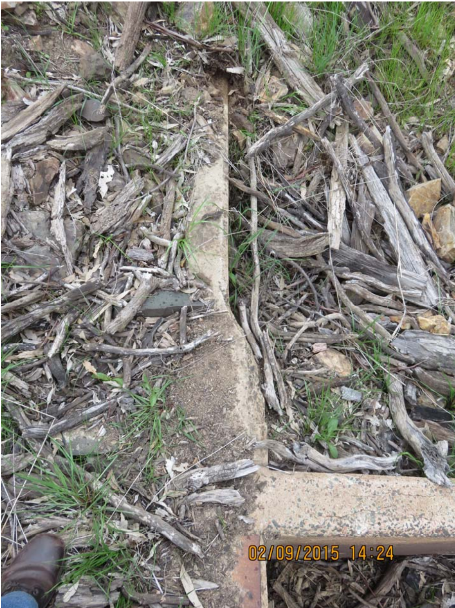
PHOTOGRAPH No.16. Note change in wall thickness on ends of headwalls.
