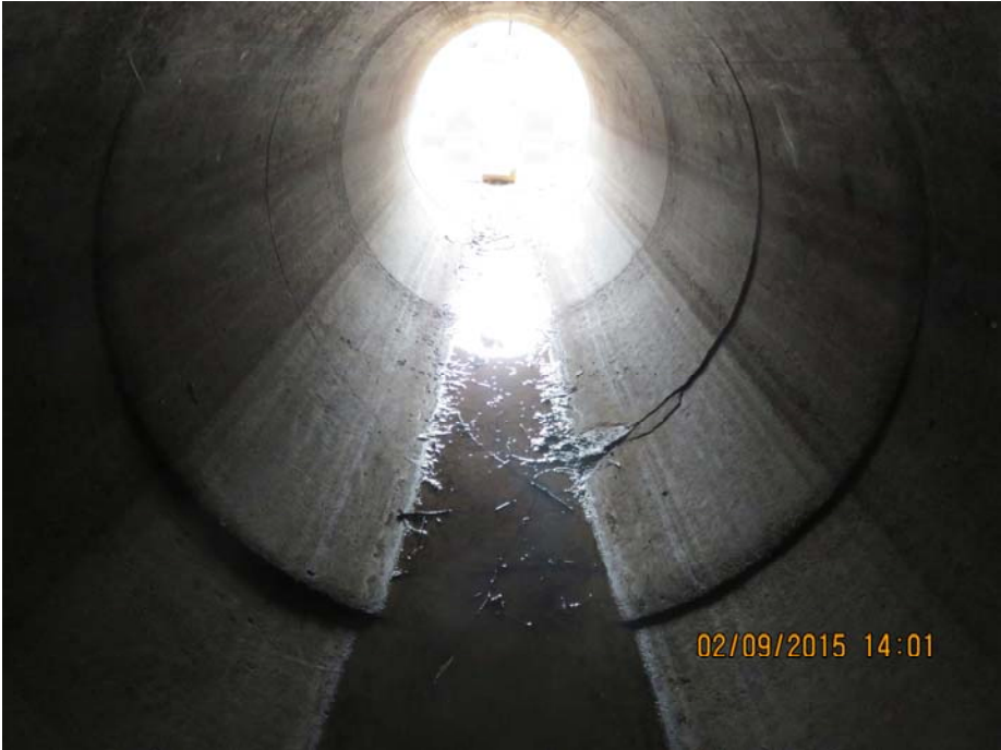
PHOTOGRAPH No.28. Dis-jointed pipe. 10. Downstream Side
