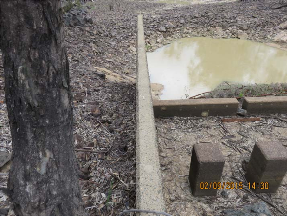
PHOTOGRAPH No.37. Wingwalls are straight.
