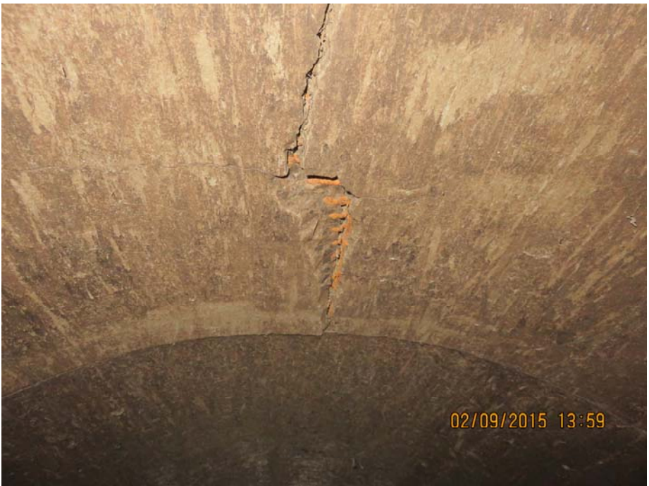
PHOTOGRAPH No.23. Exposed reinforcement.
