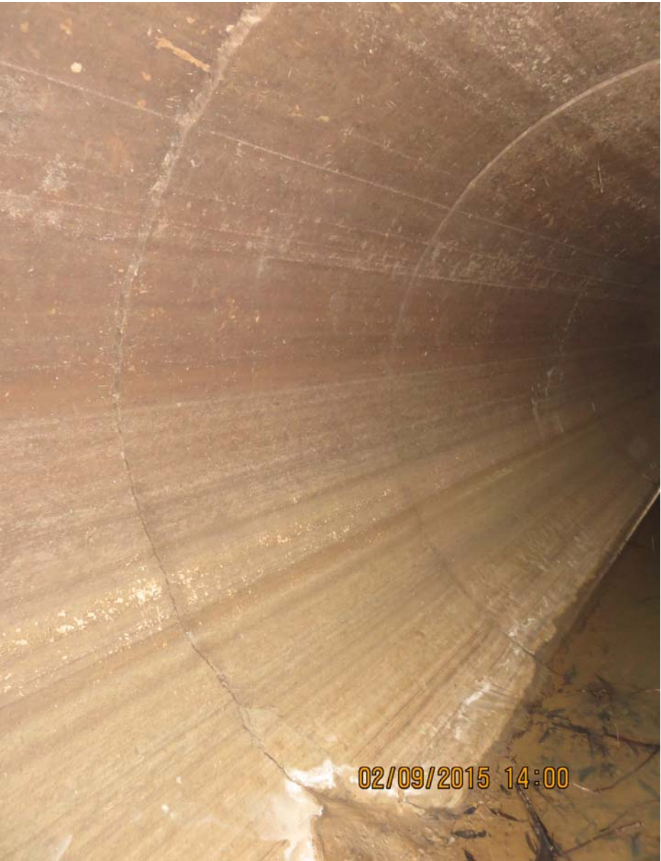
PHOTOGRAPH No.27. Dis-jointed pipe.
