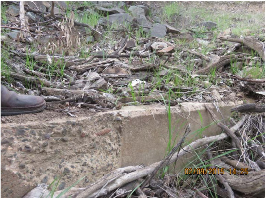
PHOTOGRAPH No.17. Machine damage to headwall.
