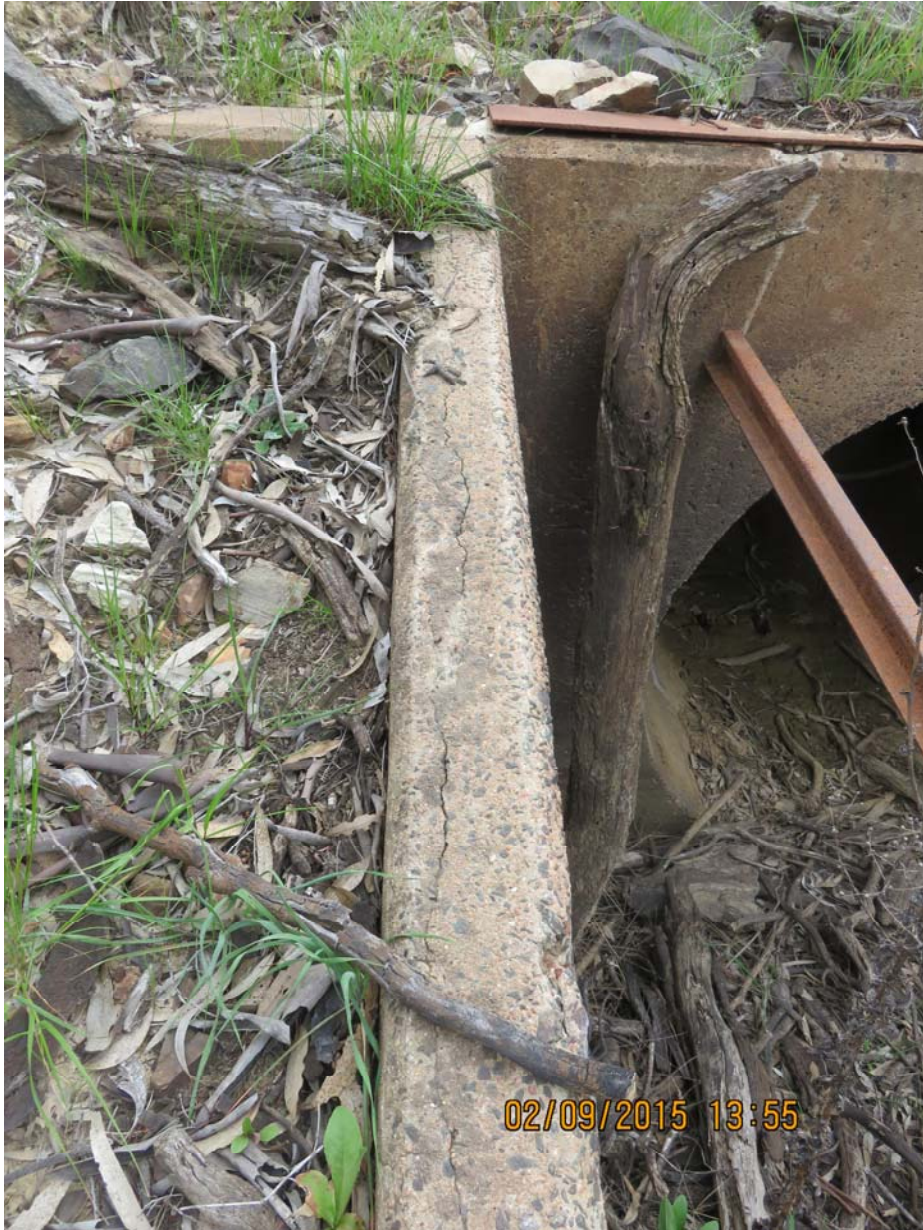
PHOTOGRAPH No.9. Note longitudinal cracks along top of wingwalls.
