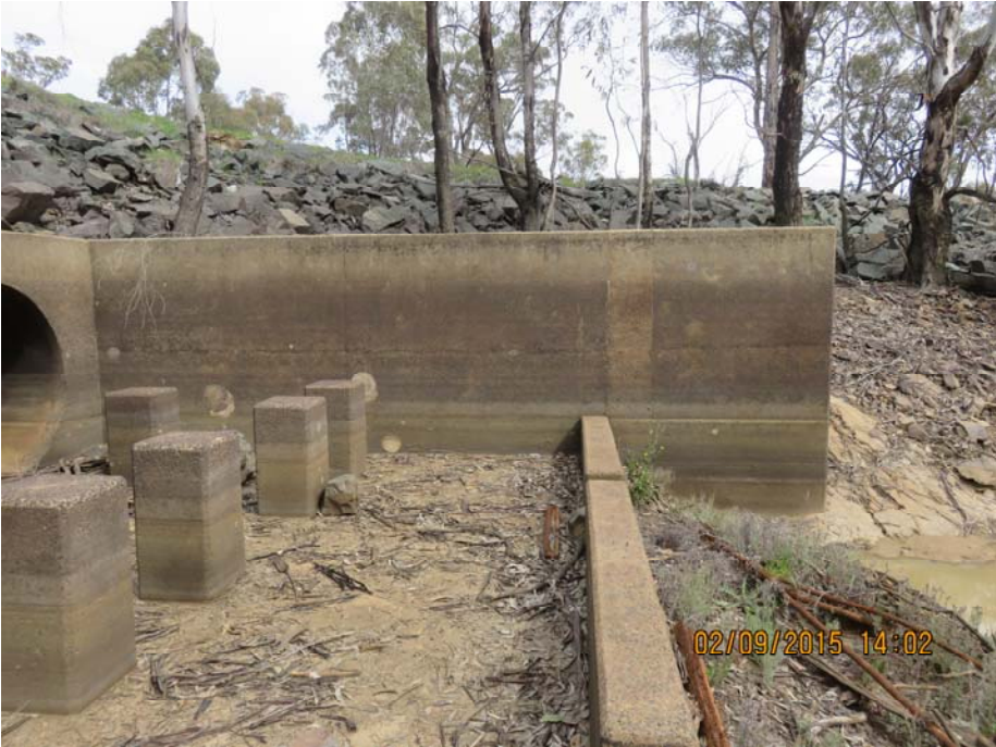
PHOTOGRAPH No.31. Note severe erosion below kerb.
