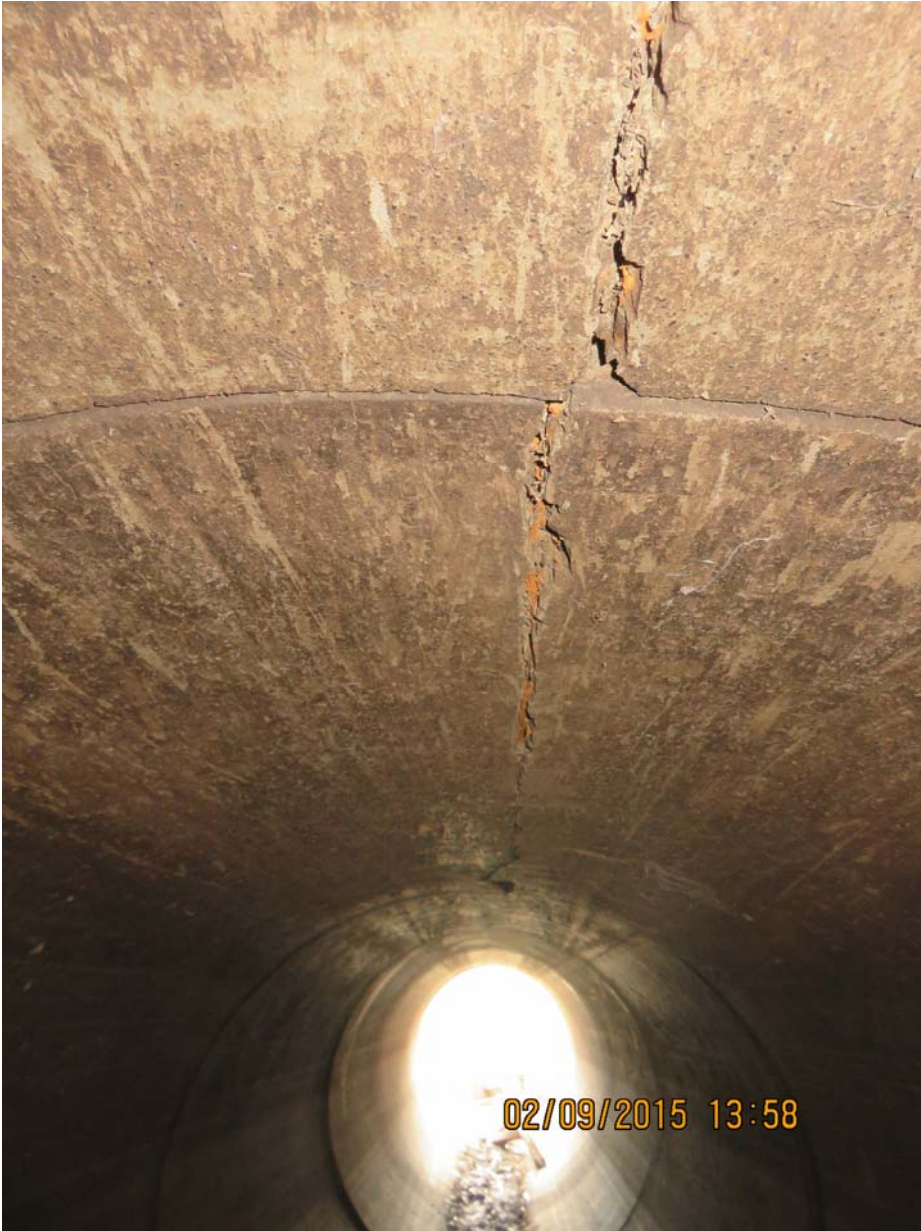
PHOTOGRAPH No.22. Longitudinal fracture in obvert of pipes.
