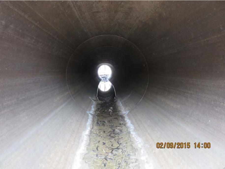
PHOTOGRAPH No.26. Dis-jointed pipe. 9. 1650 Dia. Pipe – from Downstream End
