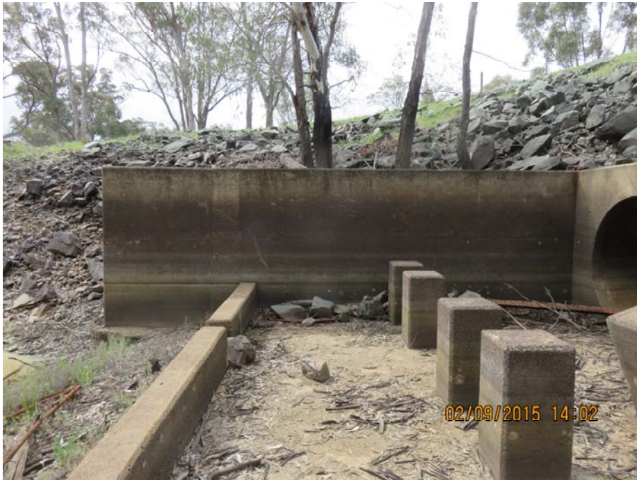
PHOTOGRAPH No.32. Note narrow kerb slots, 2 slots only 200mm wide.
