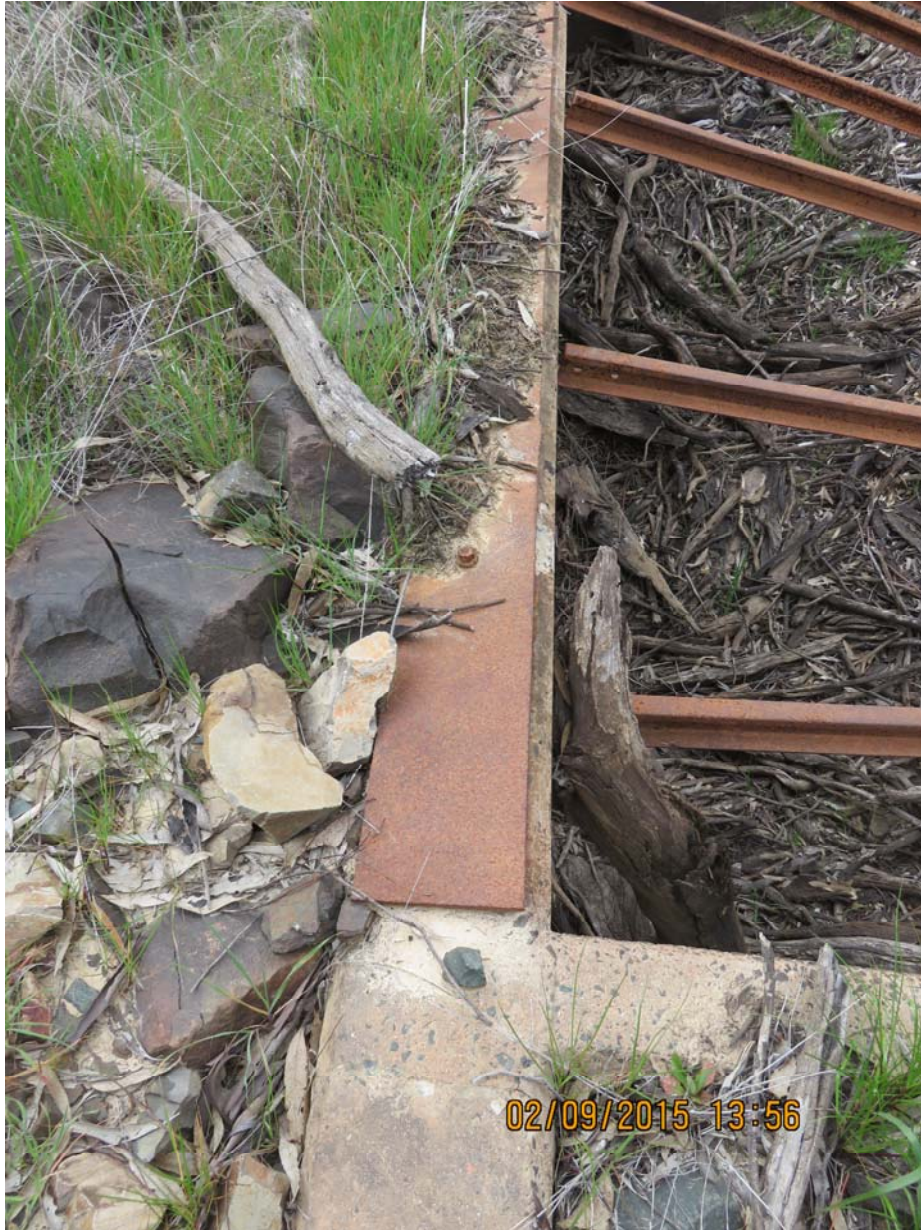
PHOTOGRAPH No.11. Note trash rack rails not attached to headwall?
