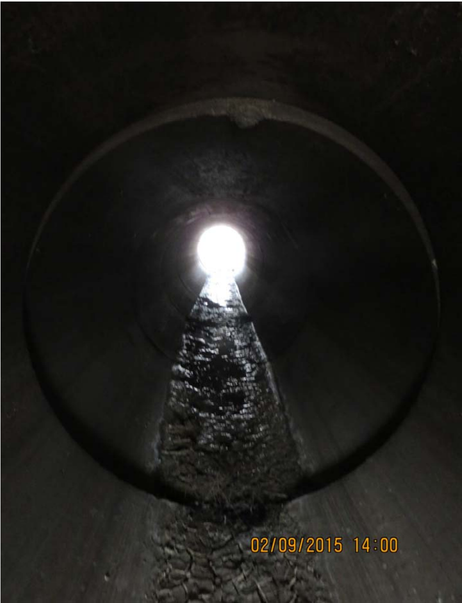
PHOTOGRAPH No.25. Dis-jointed pipe.
