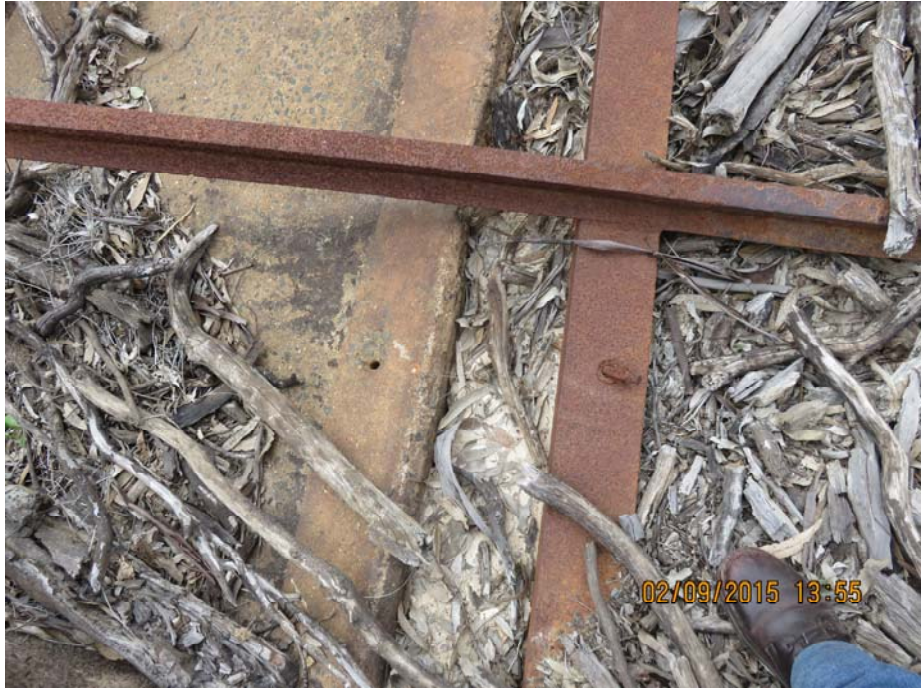
PHOTOGRAPH No.10. Trash rack fixings have pulled out of the apron.
