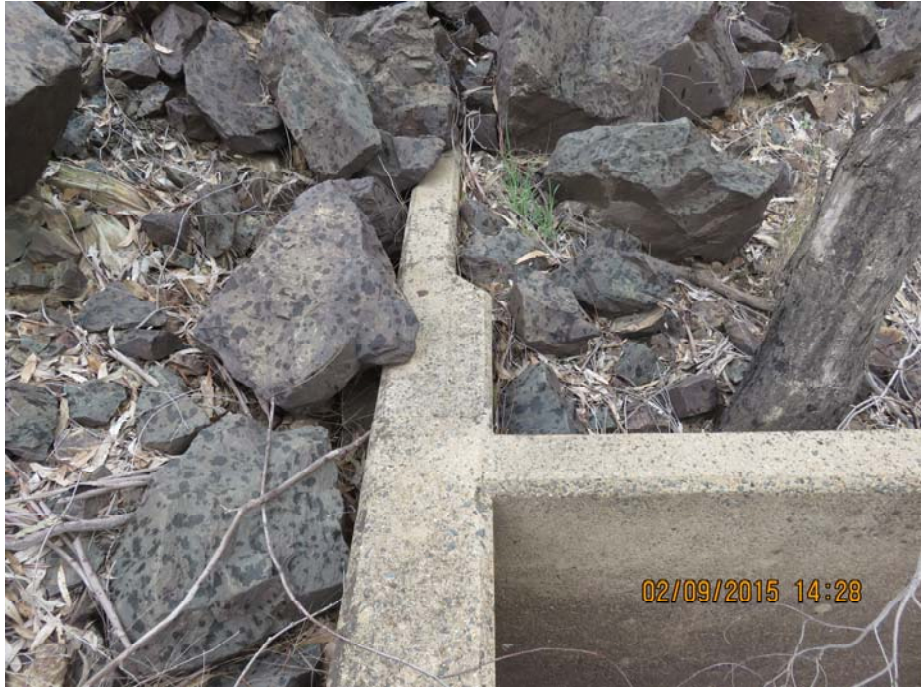
PHOTOGRAPH No.35. West side of headwall has same extension and taper.
