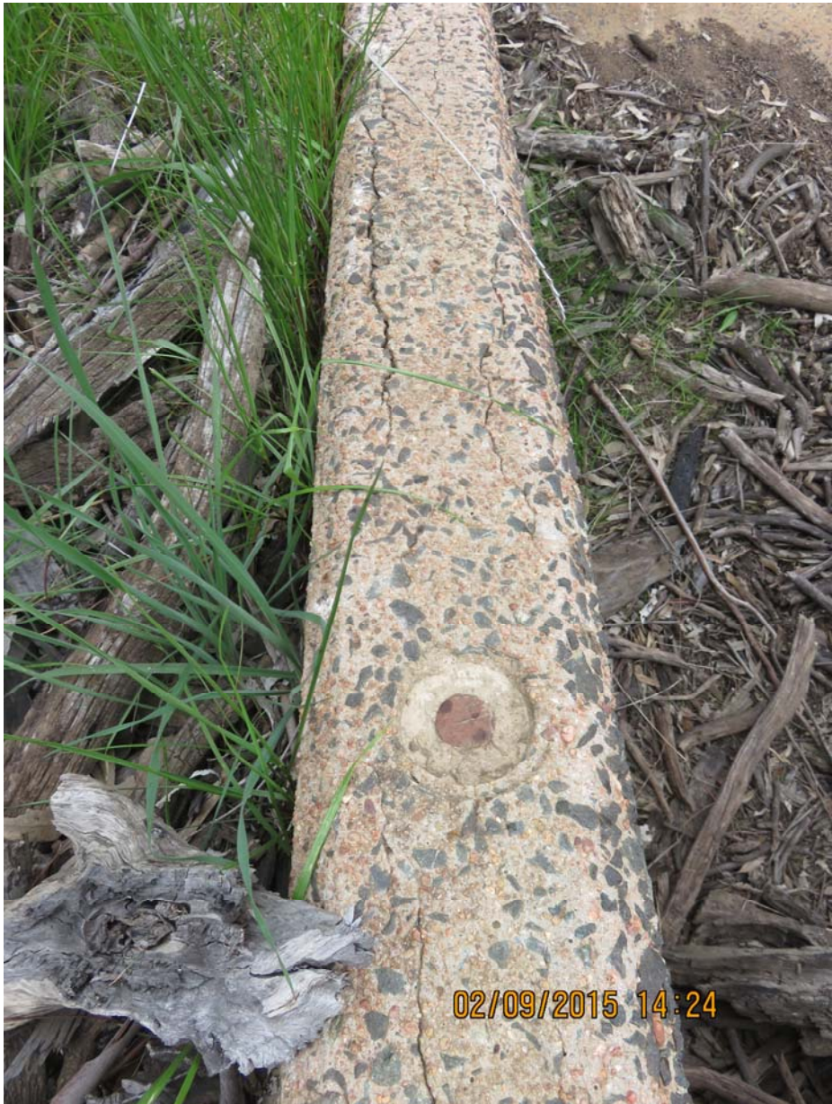
PHOTOGRAPH No.15. Longitudinal cracking in wingwalls, note lifting point?
