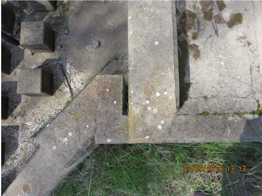
PHOTOGRAPH No.38. Looking down on abutment, wingwall deck and kerb.
