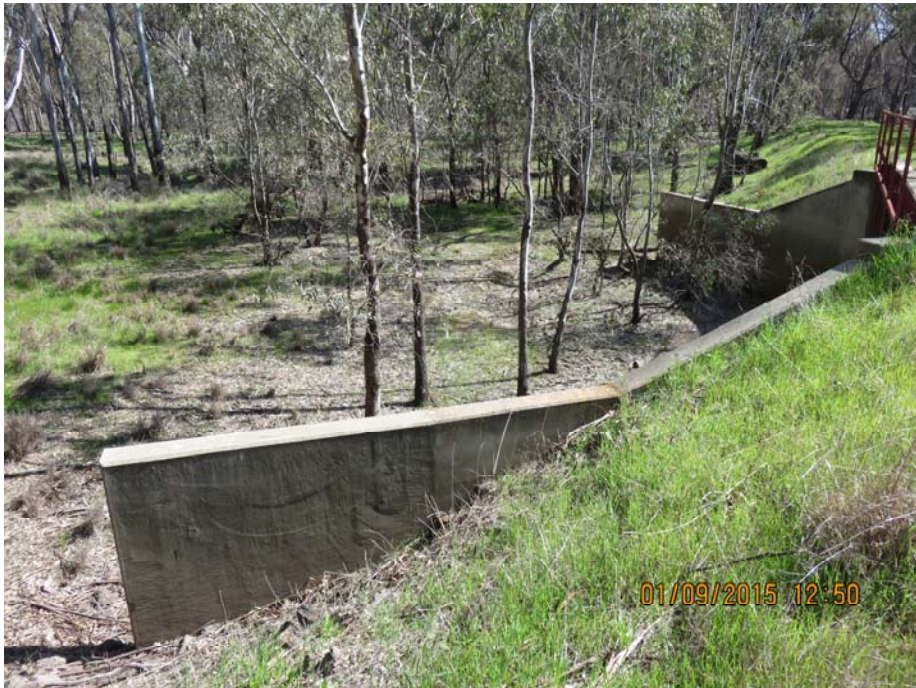
PHOTOGRAPH No.26. Looking west along upstream side.
