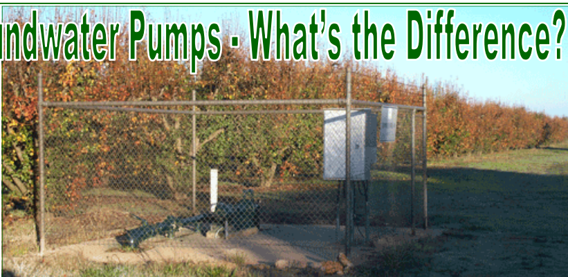
One of 43 public groundwater pumps in the SIR used to dispose of highly saline groundwater and maintain the catchment's salt balance.
