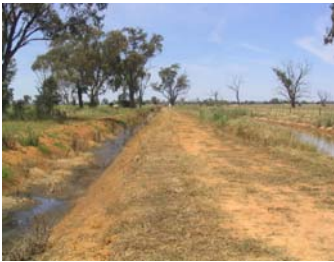
Irrigation drainage line with adjacent reuse system.
