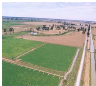
Salinity mitigation works — Muckatah Surface Water Management System
