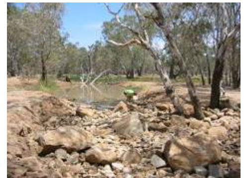
Right: Steve Collins (CMA) designed this rock chute—installed after the decommissioning of McLaughlin's Weir, to improve fish migration.
