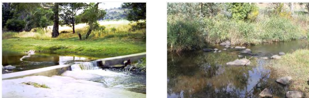
Figure 43 Left photo. Concrete weir at Hughes Creek at Tarcombe Road (No. 405228) gauging station on 27 November 1991 when the weir acted as a physical barrier to fish movement under low streamflows. Right photo. New rock ramp fishway which drowns out the original concrete weir under low streamflows on 28 April 2014.
