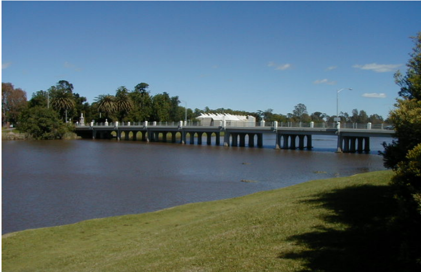
Broken River / Lake Benalla River reach of significant social and economic value
