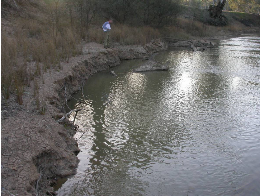
Figure 18: Notching at the toe of the bank possibly related to the long-duration IVT of summer 2006 (Reach 5, view downstream).
